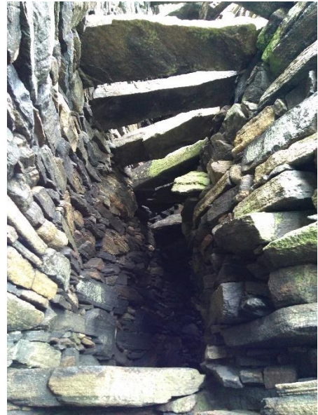
Image 2: Wall cavity with internal steps
